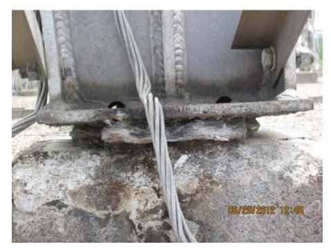
Figure 1: Example of Aluminum Oxide Formation between Concrete Surface and Aluminum Baseplate
