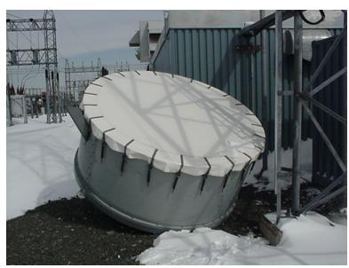
Figure 1: Microwave Antenna with Radome
