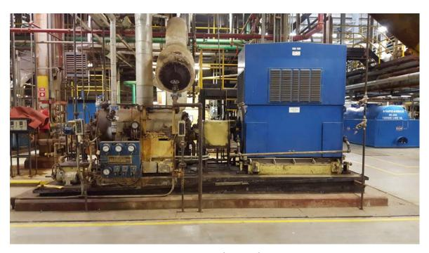
Figure 1: Unit 2 Boiler Feed Pump
