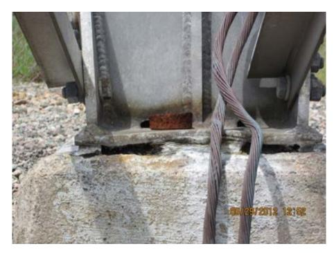
Figure 2: Example of Deformation of Baseplate Due to Aluminum Oxide Uplift
